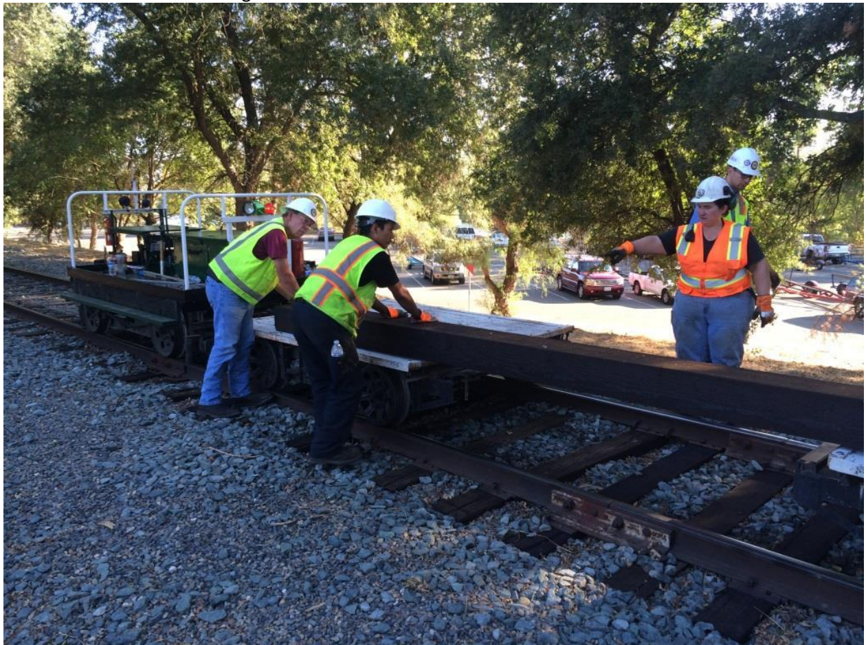
At Switch 16, Heather demonstrates the proper supervisory stance
