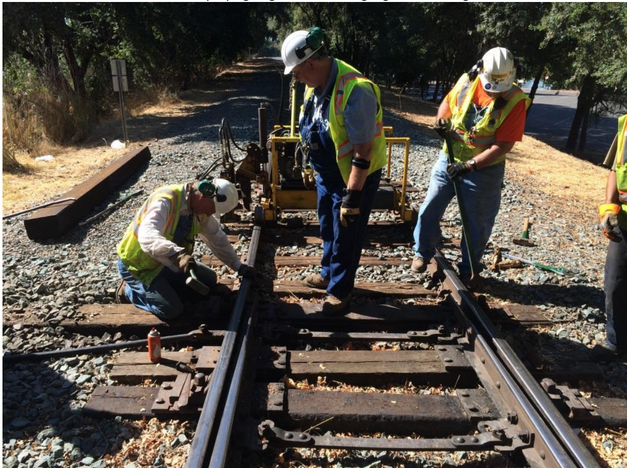
Reality has set in. The gauge plate must be removed. Steve, Chris and Mike F. start that process
