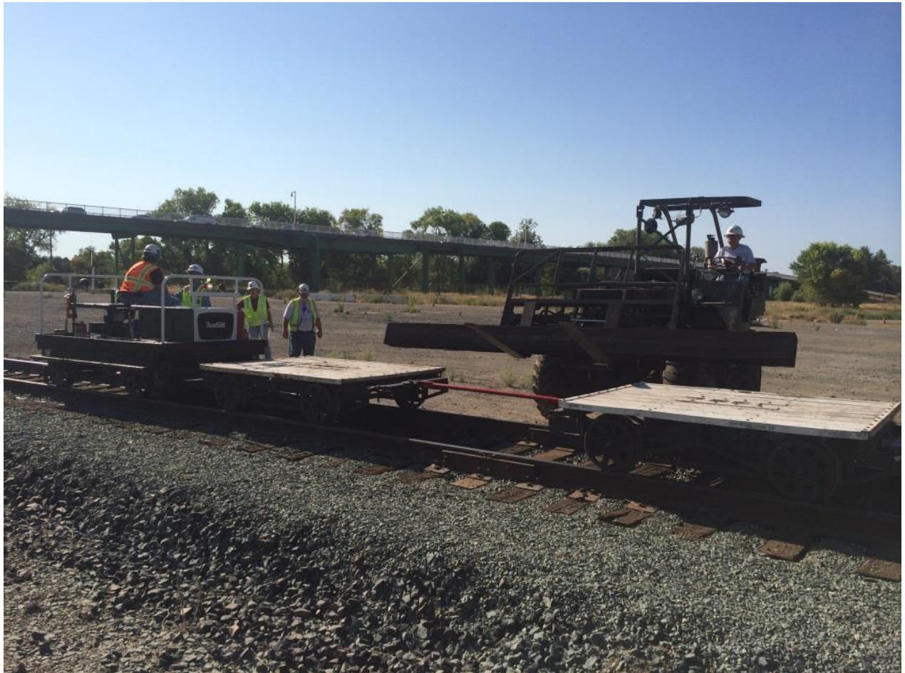
Mike H. loading the new head-block on the flatcars with the Green Machine
