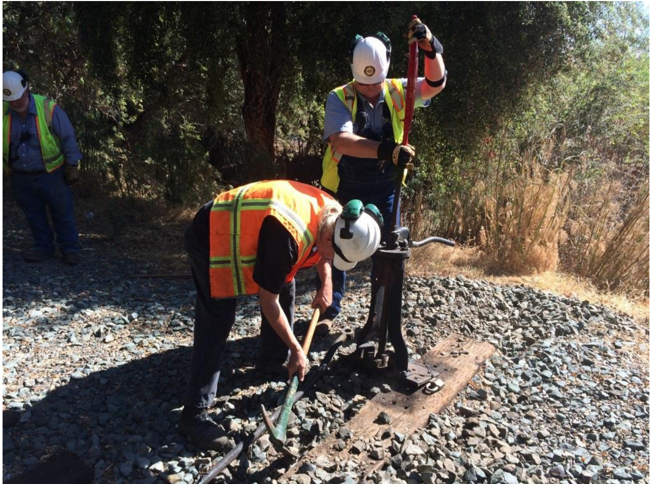
Chris and Fred work to reconnect the switch machine
