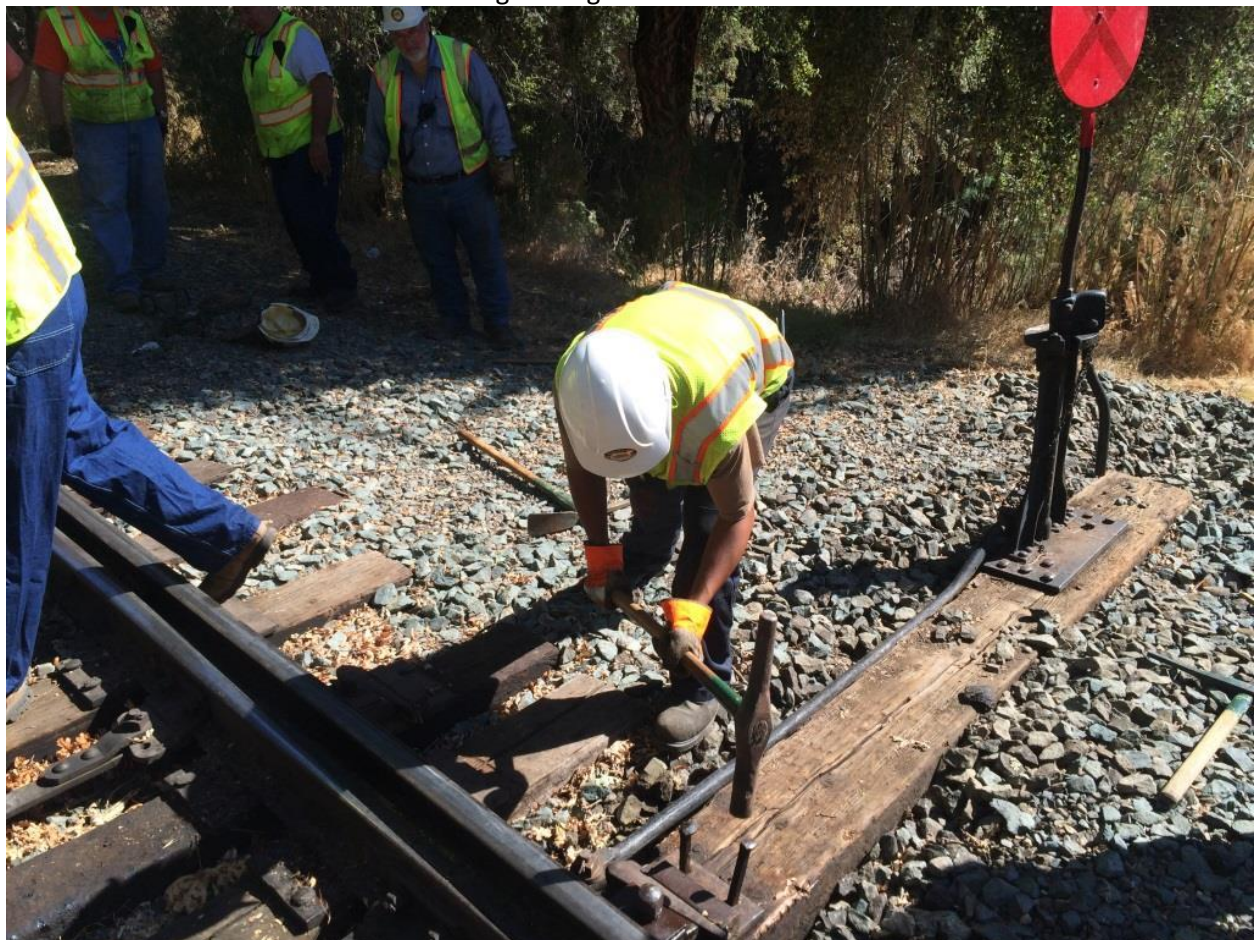
...and Josh pounding down the last spikes in the reassembly of the switch
