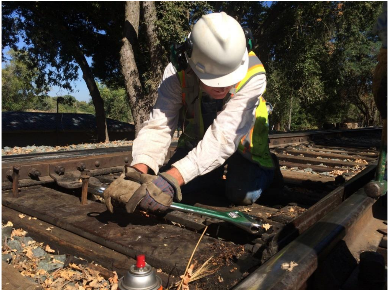
Steve tightening down the final bolt...
